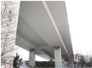
Damage to concrete bridges caused by rust can have fatal consequences, at worst leading to a total collapse. Now, researchers have developed an early-warning system for rust. Sensor-transponders integrated in the concrete allow the extent of corrosion to be measured.
